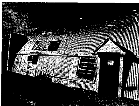
Figure 12 Side entrance for African-Americans at the Quonset Auditorium that bypasses the restaurant at the front of the building. Photo by the author.
